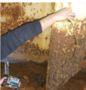
Port dock thickness measurement
